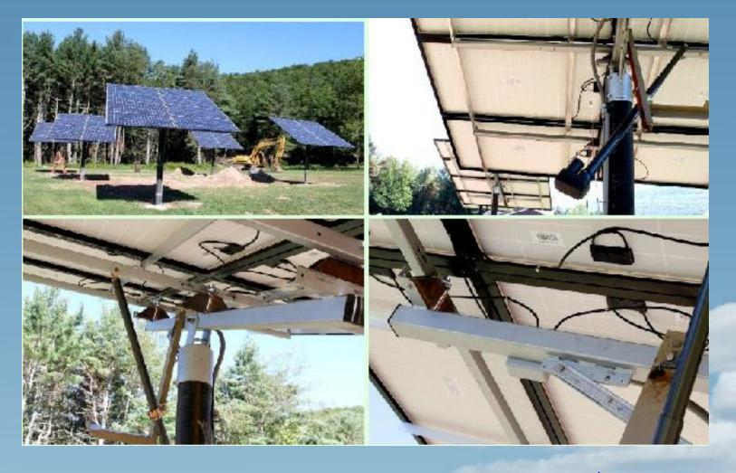
Good example of SINGLE axis tracking "ground" mount. Between \$1000 and \$2000 each, unless you're handy and trust your workmanship...
